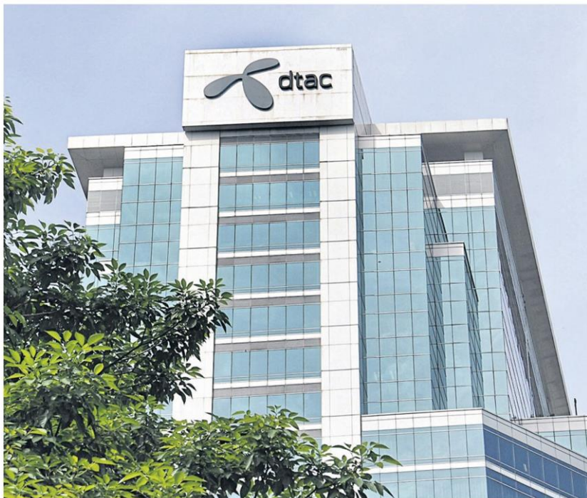
DTAC's head office at Chamchuri Square in Pathumwan district.
