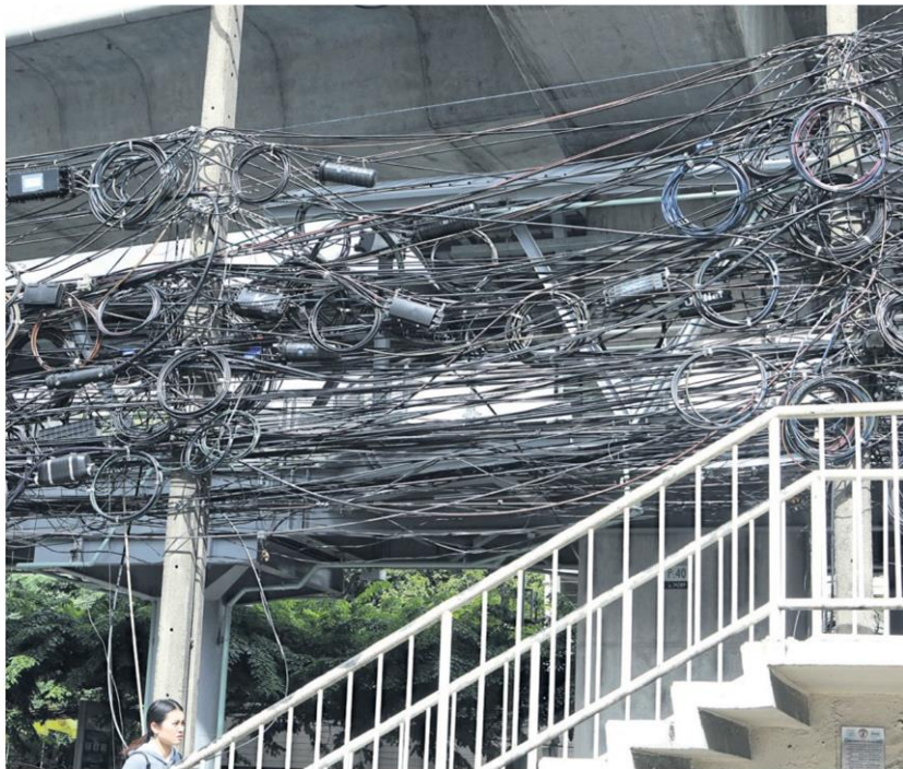
A rat's nest of cable wires hang above an overpass on Phahon Yothin Road in Bangkok. APICHIT JINAKUL
