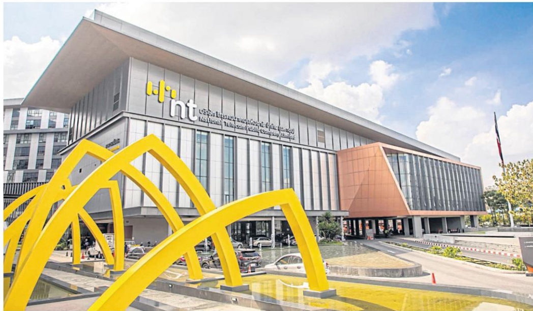
The headquarters of state enterprise National Telecom.
