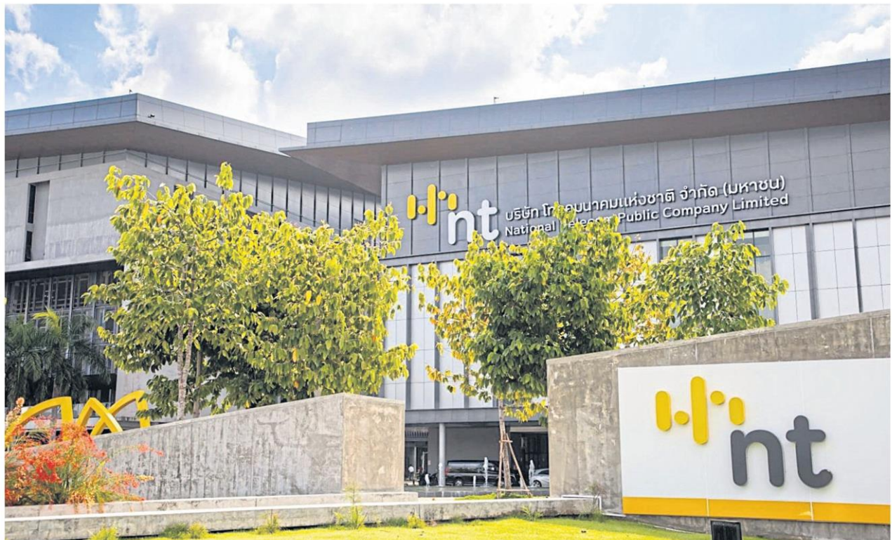
The headquarters of National Telecom, which operates a satellite business through the Thaicom 4 and Thaicom 6 satellites.
