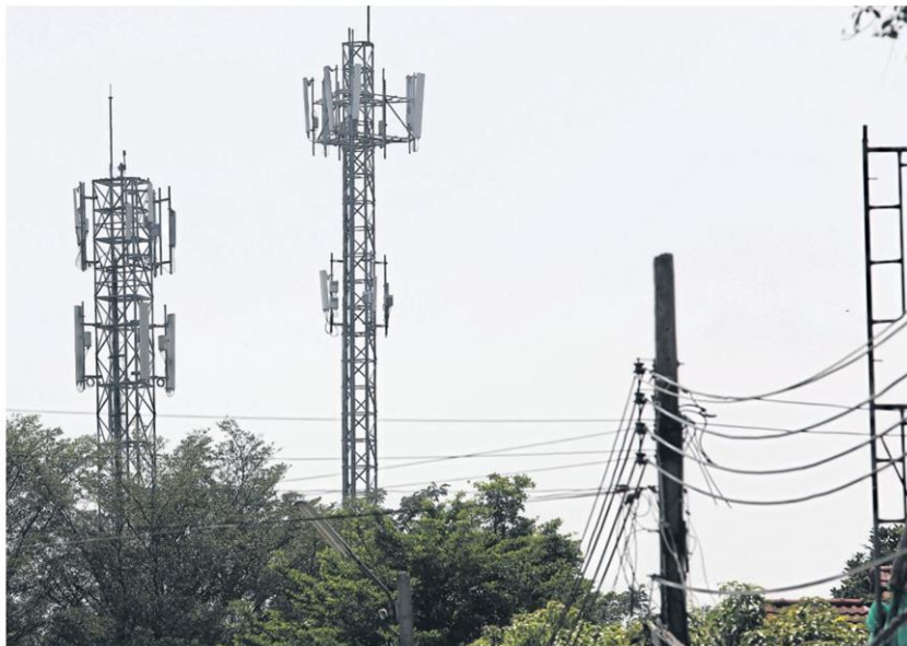
Telecom towers in a residential area of Bangkok's Sai Mai district. Locals have protested towers in their neighbourhoods over health fears. PATTANAPONG HIRUNARD
